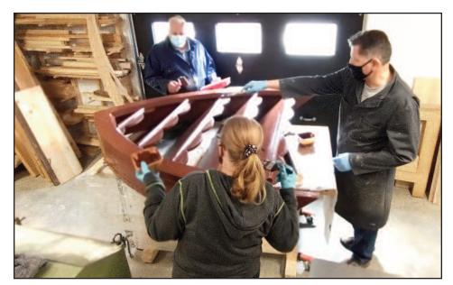
Members of MSSI assembling a louver which was built in three locking pieces for easy assembly in the church tower. Pictured front to back are: Rose, Jim and Real.
