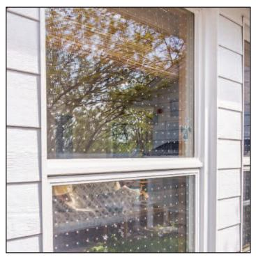
**Above:** Bird impact prevention tape is applied to the outside of windows to form a grid pattern.
